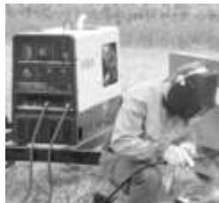
Repairing farm equipment using Hobart's Champion and 418 stick electrodes.
