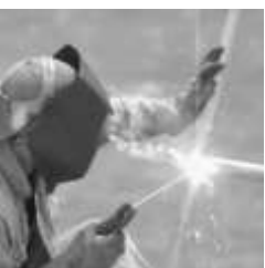
Repairing farm fencing in the field using Hobart's 418 stick electrodes
