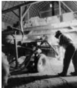
Front-end loader repair with Hobart 18AC stick electrodes
